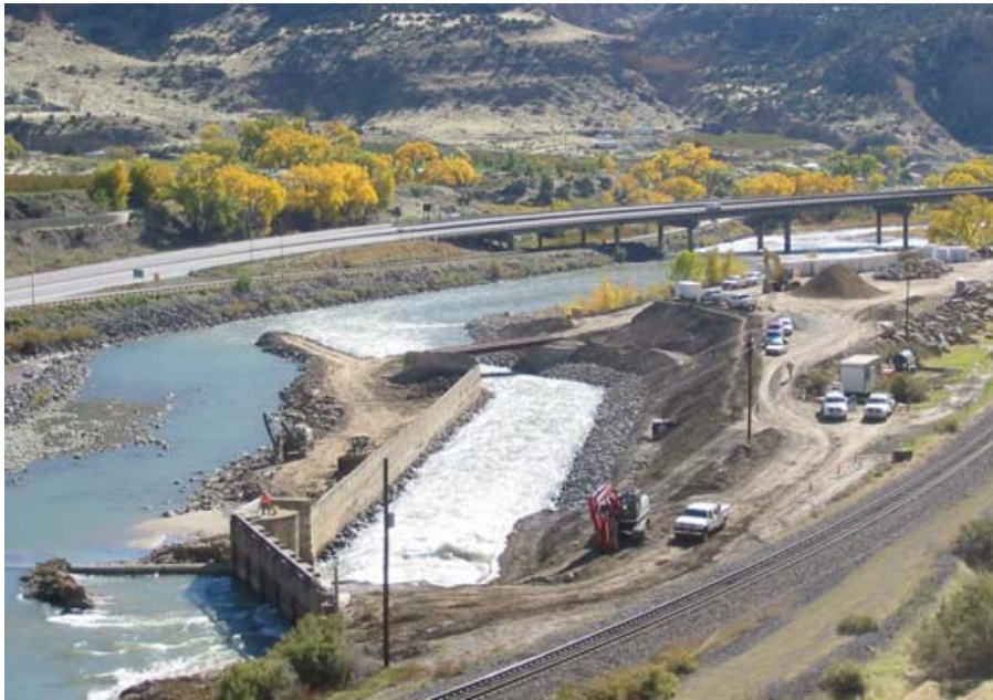
Figure 11. The Price-Stubb Diversion Dam fish passage on the Colorado River near Palisade, Colorado, was completed in 2008. Removal of this barrier to fish migration provides endangered fish access to an additional 84 km (52 miles) of critical habitat that has been blocked since 1911. Photo: U.S. Fish and Wildlife Service.
