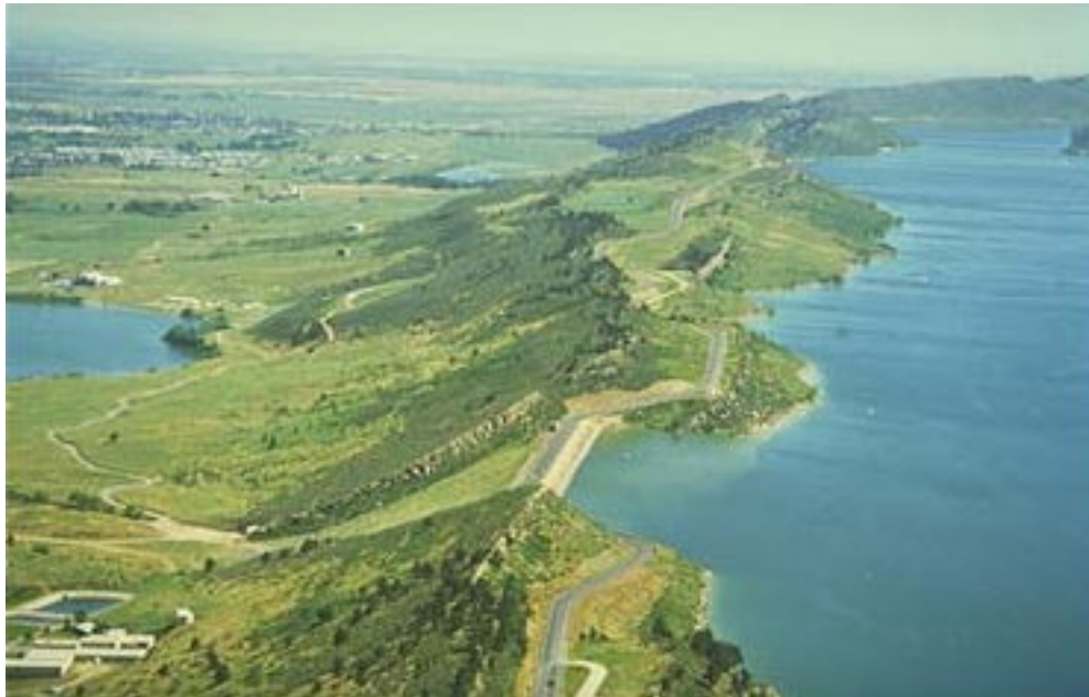
Figure 20. Horsetooth Reservoir at close to full pool conditions (photo: City of Fort Collins).
