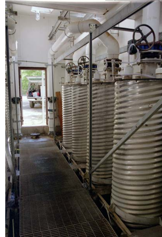
Figure A4.2. Rifle Falls Hatchery, with raceways and hatch-house pictured at left, is fed by a mix of 5 springs collected less than a mile from the hatchery. The right photo shows the area where the springs mix prior to entering the hatchery. The springs produce a consistent supply of water at a year-round temperature of 59°F.
