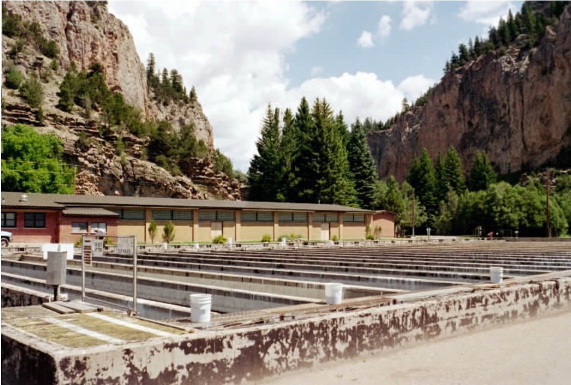
Figure A4.2. Rifle Falls Hatchery, with raceways and hatch-house pictured at left, is fed by a mix of 5 springs collected less than a mile from the hatchery. The right photo shows the area where the springs mix prior to entering the hatchery. The springs produce a consistent supply of water at a year-round temperature of 59°F.
